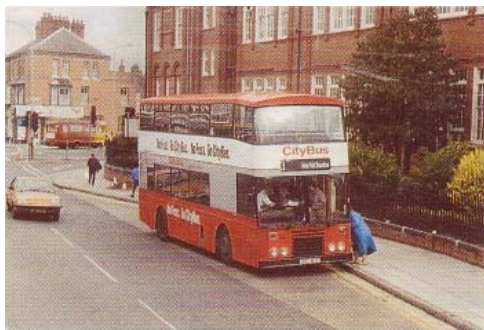
Lay-bys improve traffic flow and access to bus stops. They are best constructed in materials different from the main carriageway...
