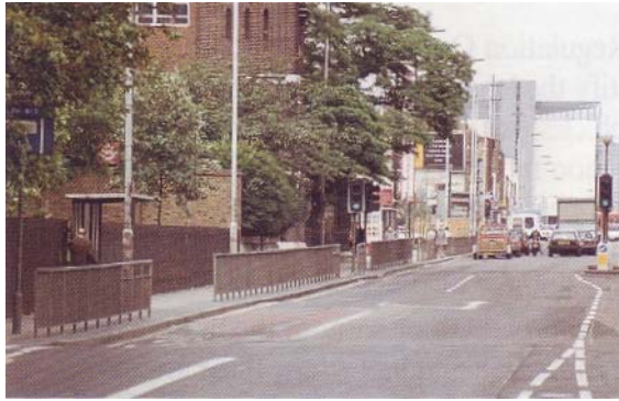
The withflow bus lane is stopped short of the signal stop line to maintain saturation flow and accommodate left turns
