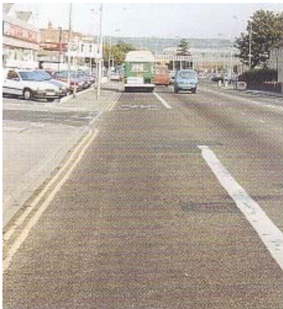
The outer edge of the bus lane should be marked by a solid white line which terminates at the entrance to or exit from a side road
